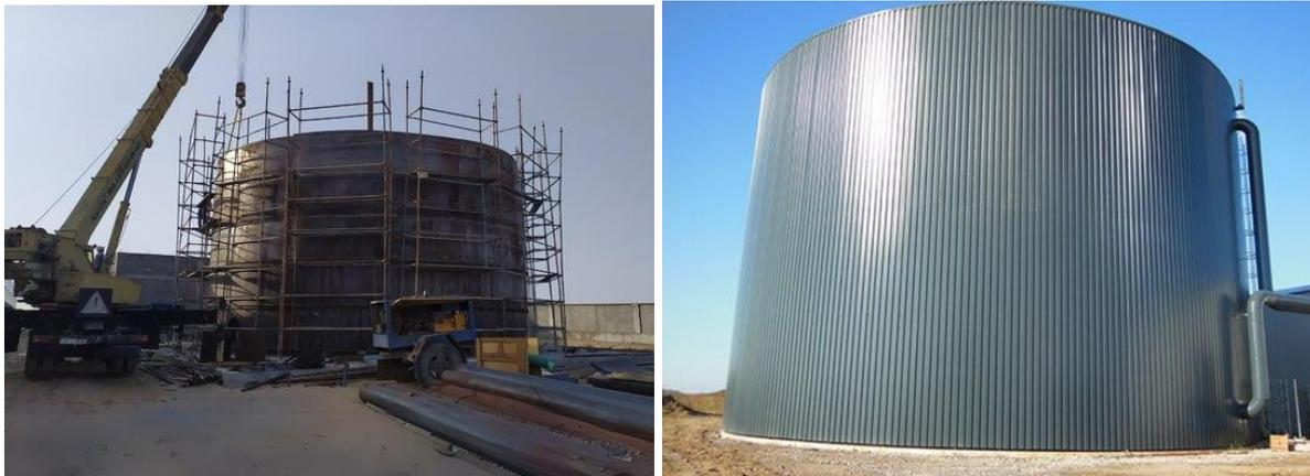
Figure 2. Cuve sans pression ou "open buffer" (source : <https://www.greenclimate.com.tr>)
