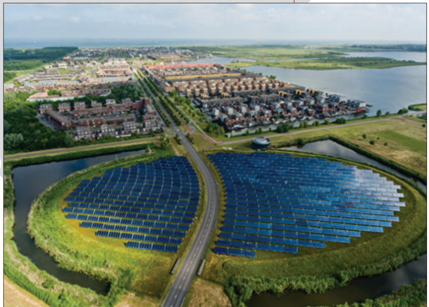
▲ The 7,000 m2 solar thermal collector field on Zoneiland Almere (Almere Solar Island) is one of the largest of its kind in the world. (Source is Nuon Vattenfall)
