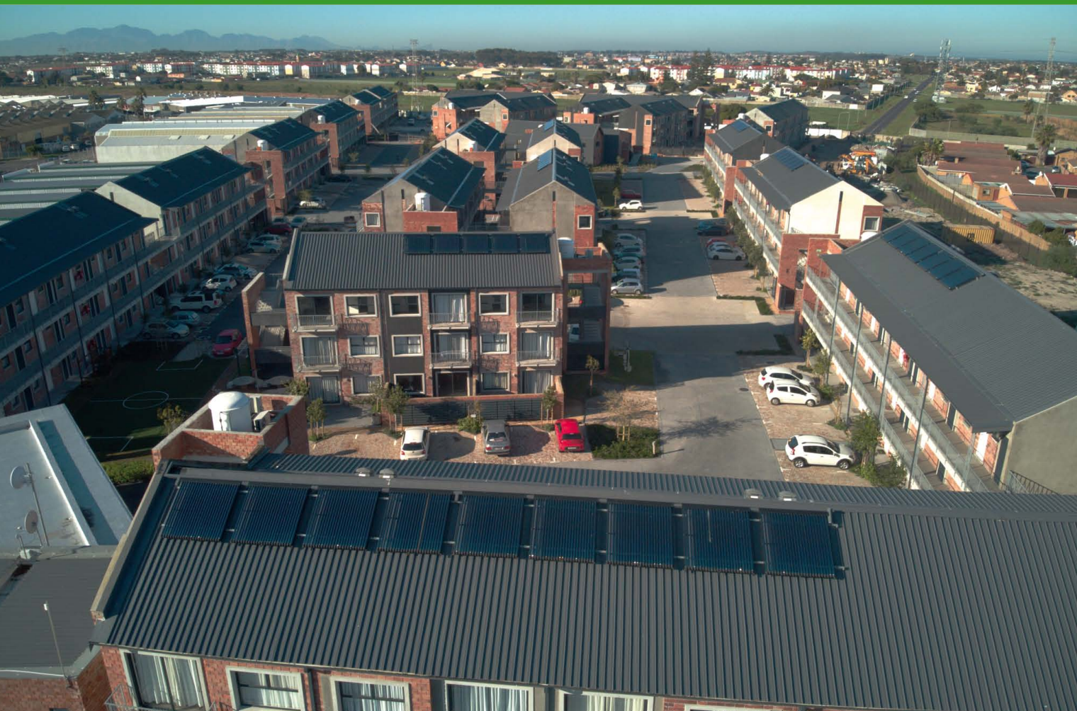
Solar water heating systems in combination with heat pumps for apartment buildings in Cape Town, South Africa.
