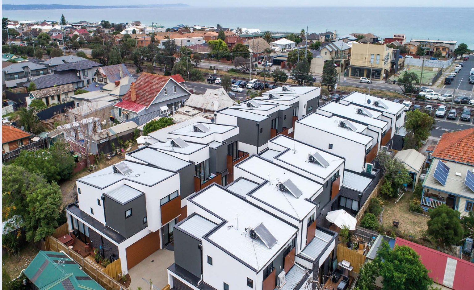
Thermosiphon systems for a neighborhood in Station St Edithvale, Australia.
