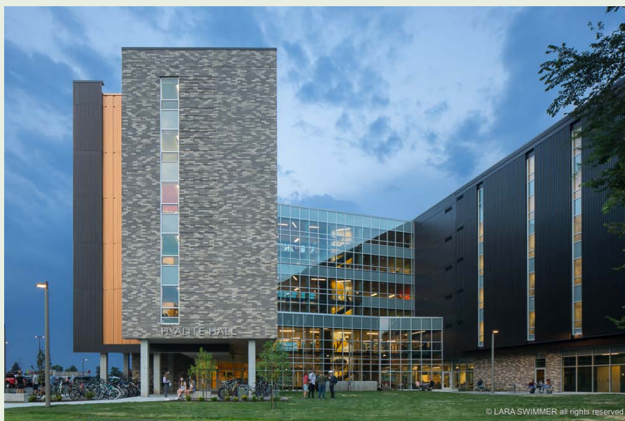
0.6 MW th façade integrated solar air system at Hyalite Hall, Montana State University, Bozeman, USA.
