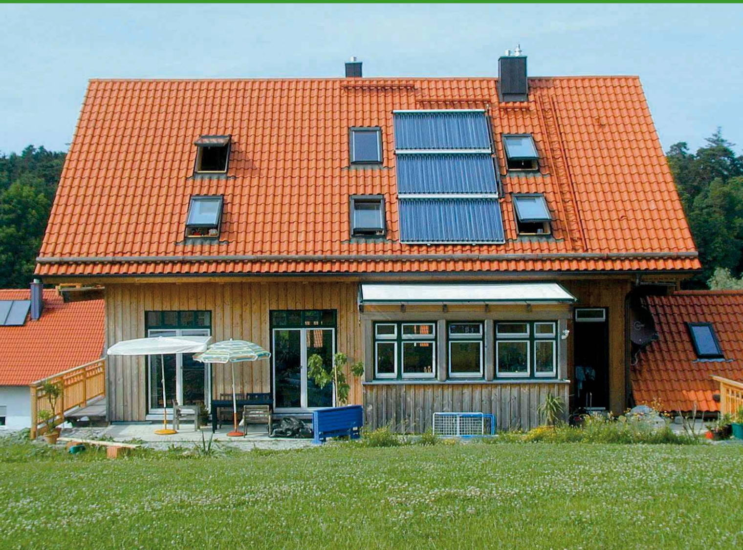
Single-family house with evacuated tube collectors in Germany.
