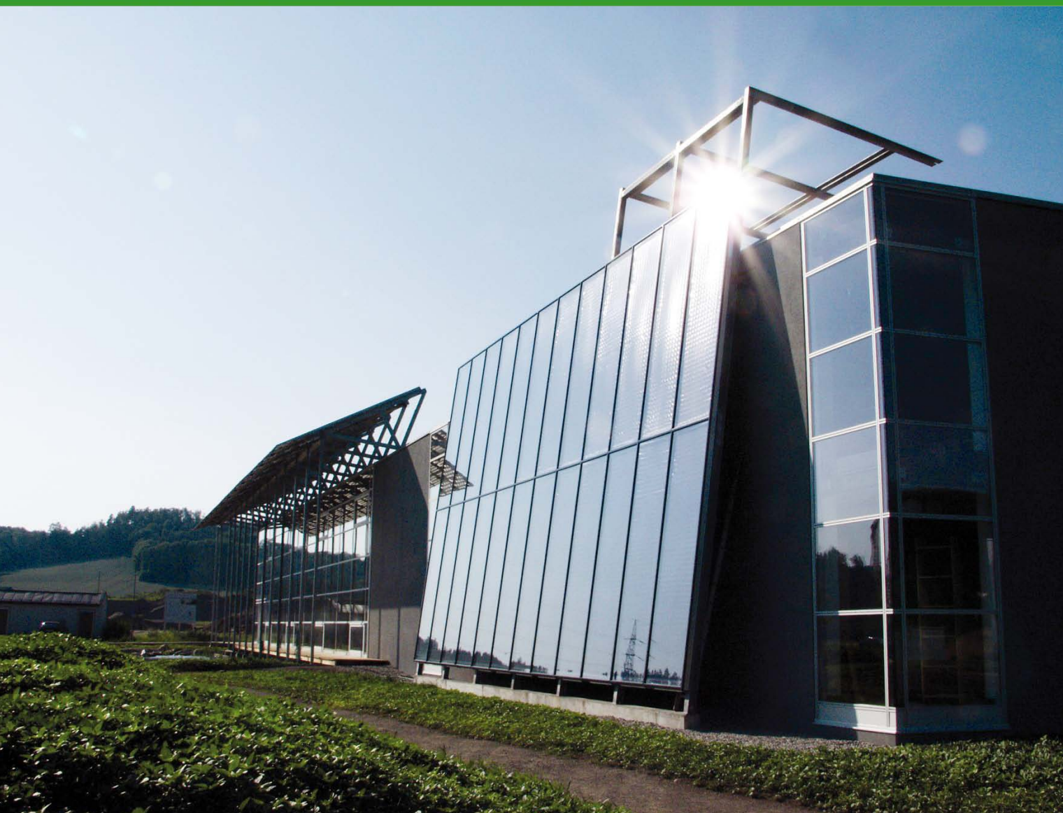
Facade-integrated collectors in St. Veit, Austria.
